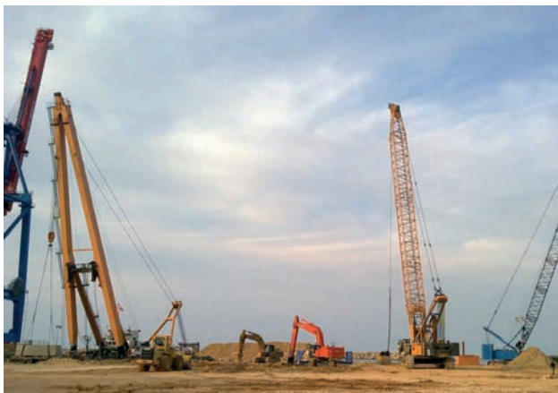
Cranes at work: floating crane, dynamic compaction, piling crane.
